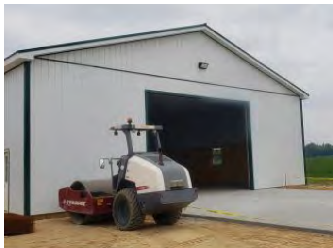
One of two new pole barns constructed for the wood products business and partially funded by the MARBIDCO WPIEI grant.
